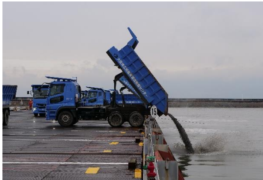
Photo 2-12 The Dumping of Waste into the Landfill (Reclaimed Land off Osaka Coast)
