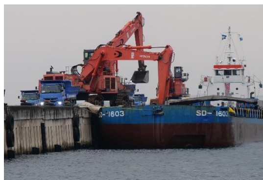
Photo 2-11 Transfer of Waste from Ship to Truck (Reclaimed Land off Osaka Coast)
